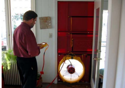
Performing a Blower Door Test for air infiltration
